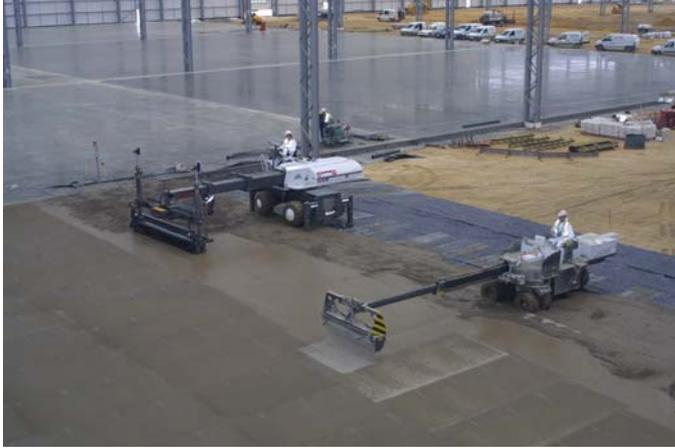
Mechanised large bay construction using the Somero SXP® Laser Screed® allows very large areas to be cast as a single continuous pour, thereby eliminating the need for construction joints. With constant reference to a laser level, surface tolerances are optimised and are uniform in all directions. Whether in the UK, Europe or the United States, there is rarely a large industrial concrete floor being poured these days without the use
